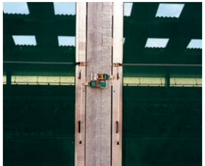
Ratchets ensure firm tensioning even in high winds
