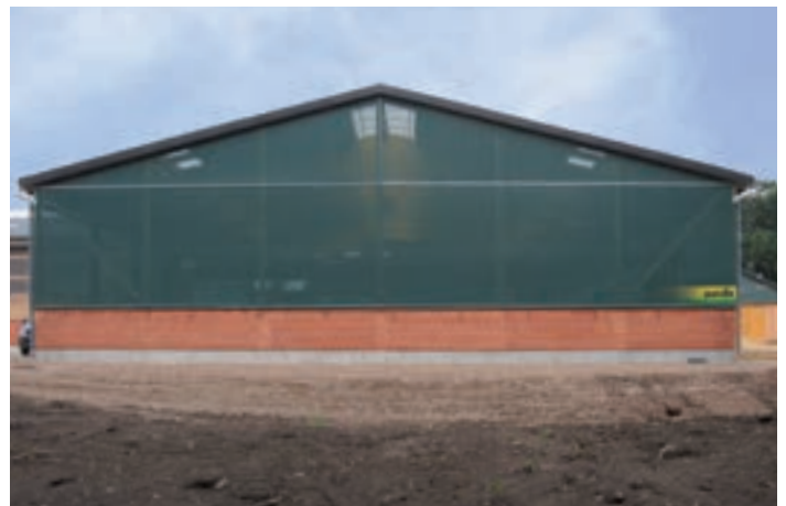
Fixed system with kador profile on top and laid-flat pocket at the bottom. Tensioning via steel tubing (in the laid-flat pocket) and ratchets
