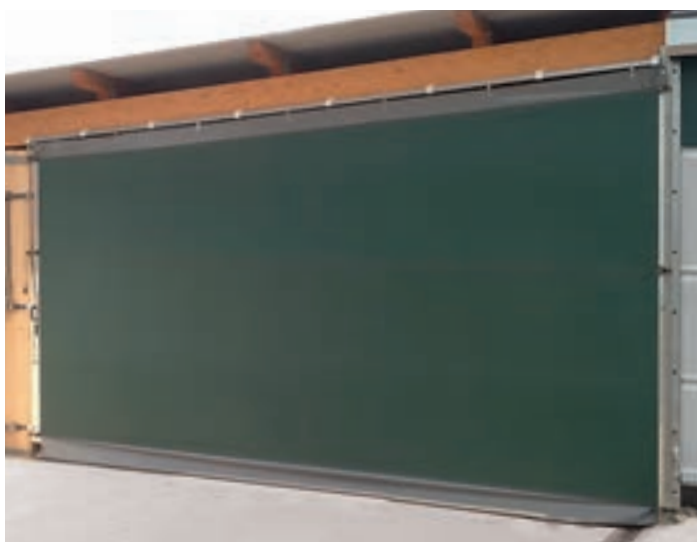
Trackscreen curtains for optimal light and climate conditions, the complete front of the indoor riding ring can be opened by sliding the curtain to one side
