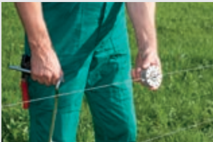
1. Place the rotating wire tensioner on the wire, attach the wire tensioner handle
