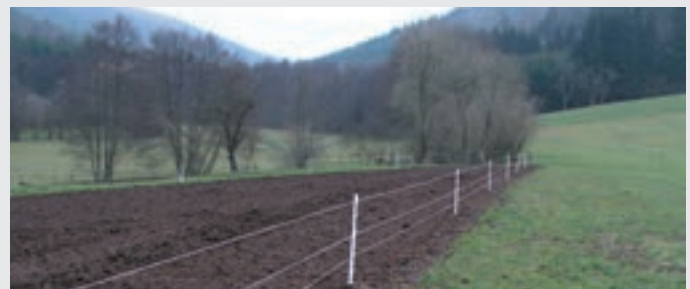
In just a short time the electric fence is ready for use
