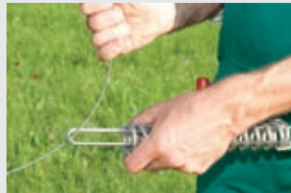
1. Thread the wire through the tug link of the tension spring
