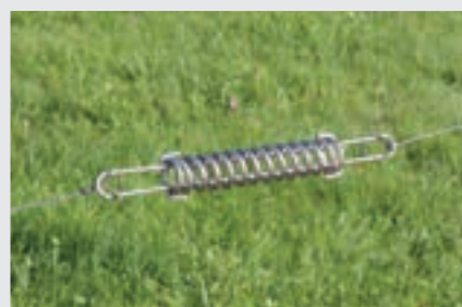
4. Repeat the fastening on the opposite side and pre-tighten the spring with the rotating wire tensioner
