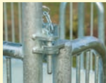
Easy-to-open side panels through socket pins
