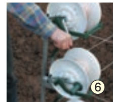
6 ... tension by winding back on the reels
