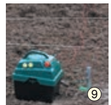
9 Attach and earth the energiser
