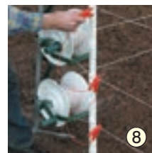
8 Attach the cross-connections approx. every 200 m
