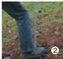
2 Set corner posts at all corners and curves
