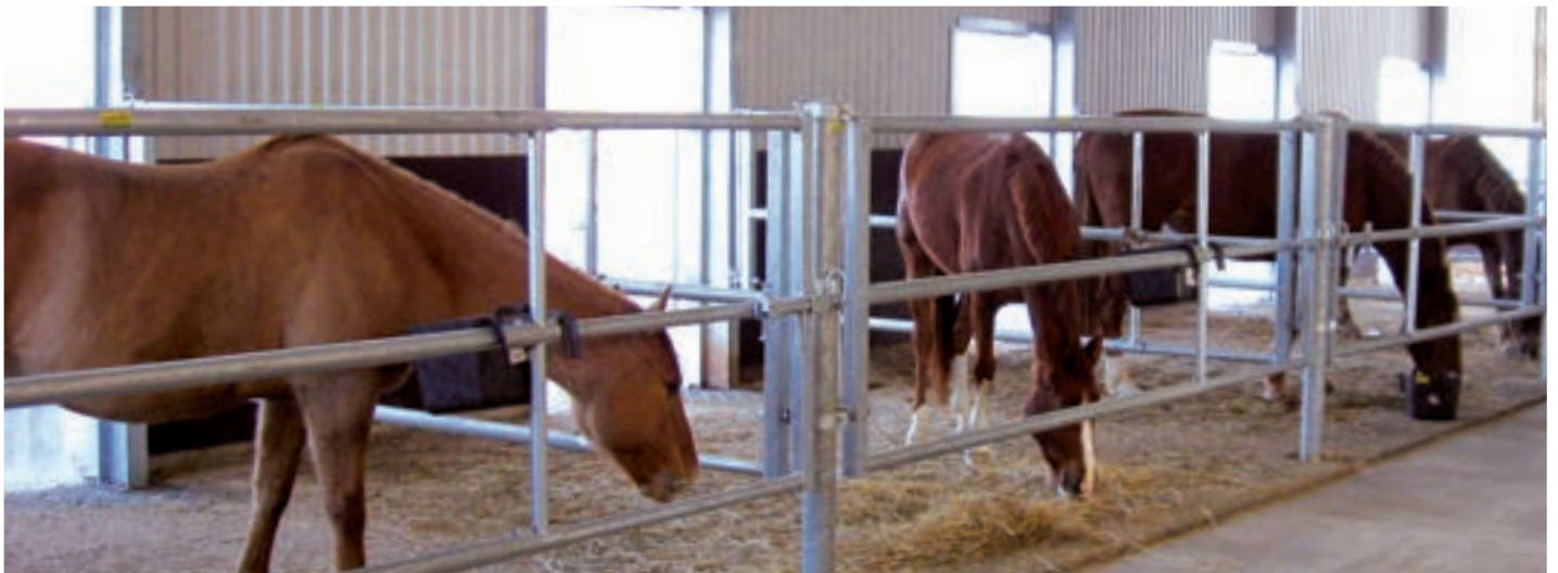
Open, low partitions for easy social contact between each other. Generous box stall dimensions (3 x 4 m) for optimal free moving space
