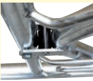
Internal plastic buffer for resetting of yoke
